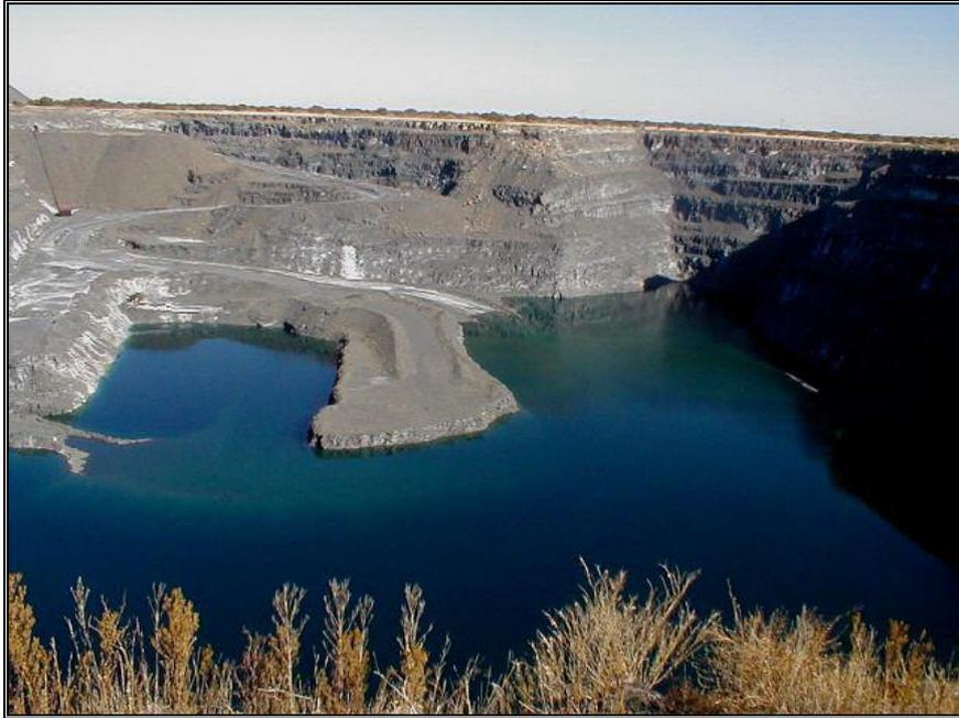
The Open cast mine at Pering. Now closed and partly filled with sulphurous water. White sulphate efflorescence developing from acid mine drainage seeping out from the open pit walls can be seen in the distance
